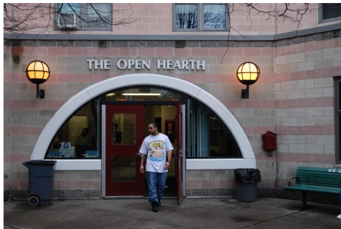
Main Entrance at 150 Charter Oak Ave. Hartford, CT
